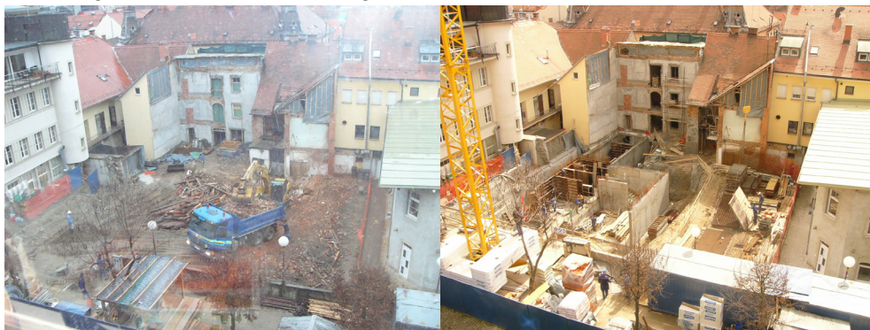
Figure 1a-b: Construction site on Gregorciceva, Maribor (SI), Author: Daniela Dvornik Perhavec.
