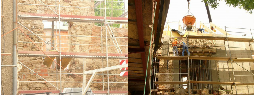
Figure 2a-b: Construction site on Vetrinjska, Maribor (SI), Author: Daniela Dvornik Perhavec.
